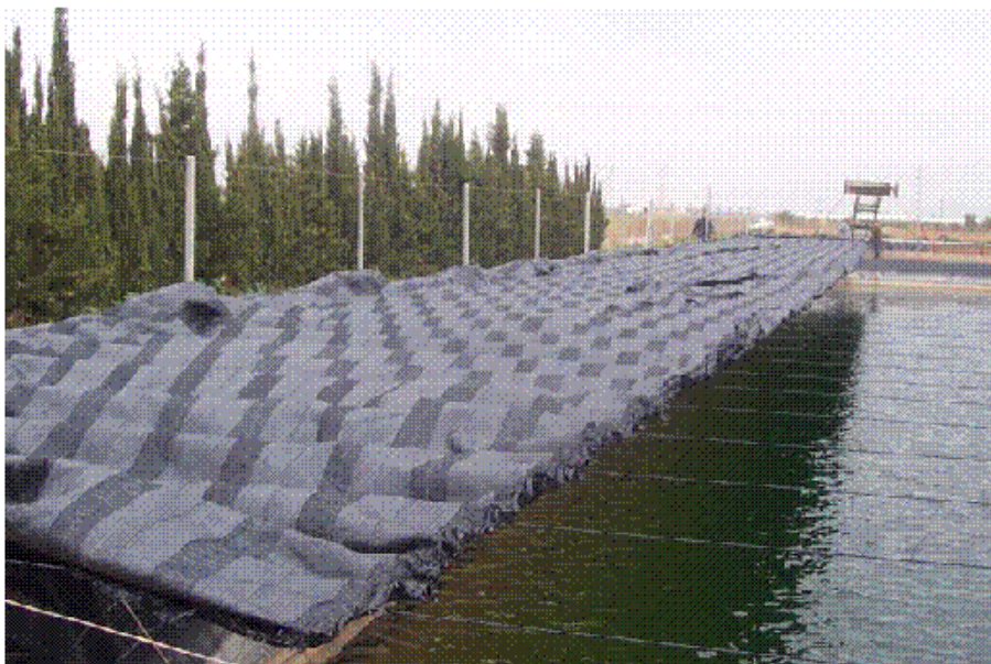
Figure 4. Installation process of the suspended cover in the experimental reservoir
